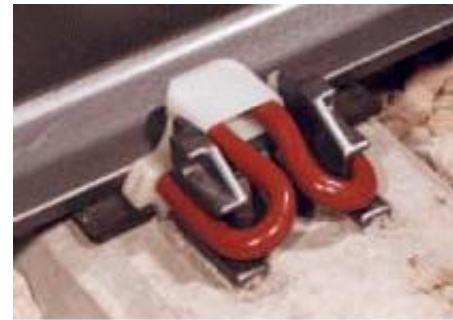
[그림] Pandrol Fastclip
