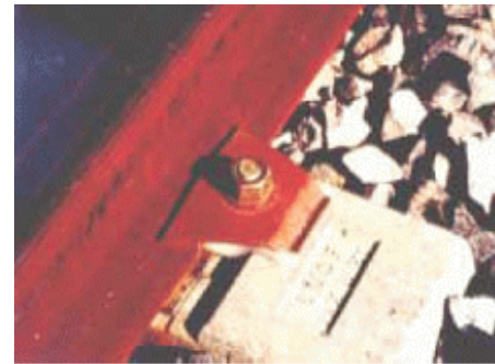
[그림] Nabla Fastening System
